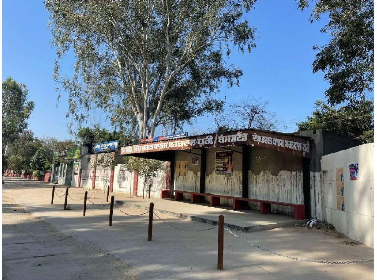
Secured Boundary walls
